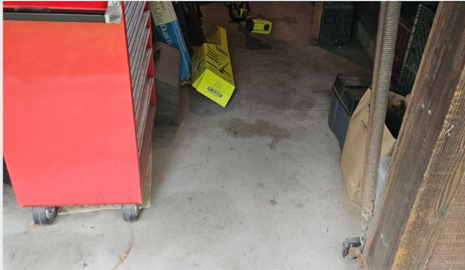
Figure 21. Garage Concrete Slab
