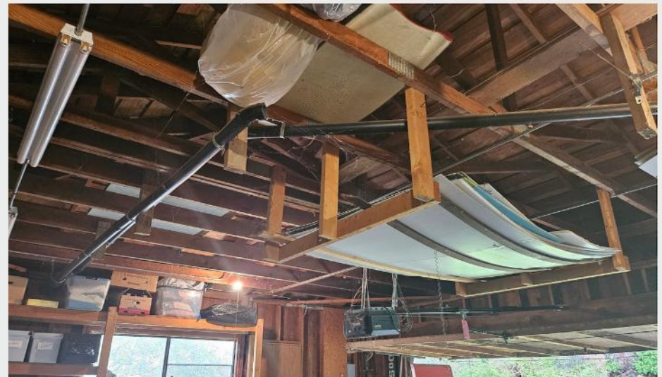
Figure 12. Garage Ceiling Structure
