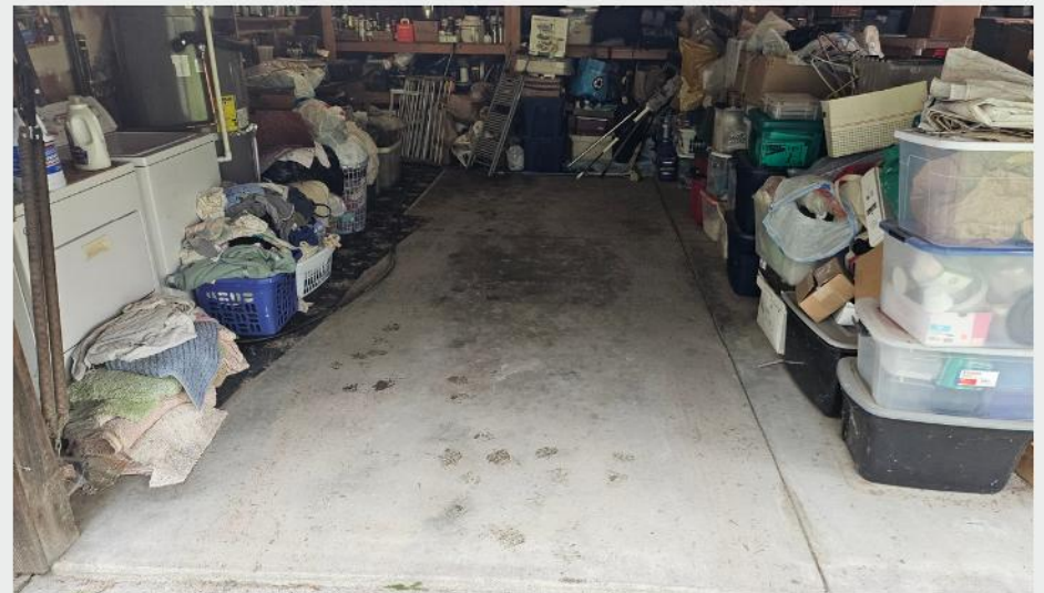
Figure 20. Garage Concrete Slab
