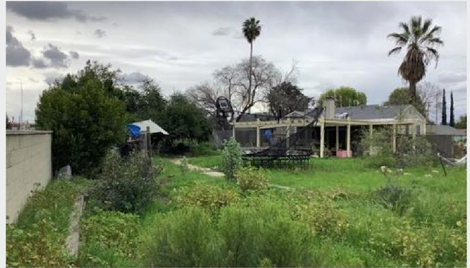
Figure 14. Backyard from Lot Line
