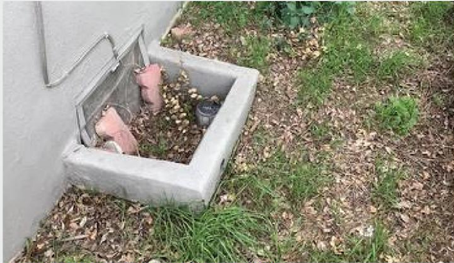
Figure 17. Nearest Sewer Point to ADU
