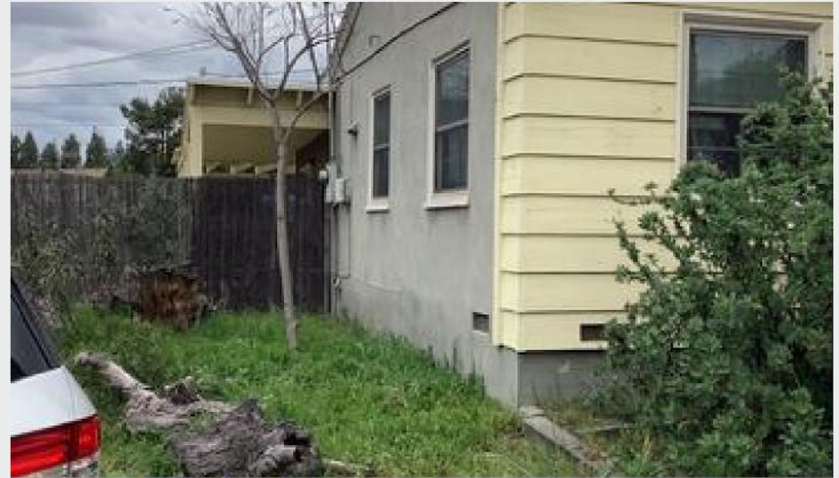
Figure 18. Electric Panel Location
