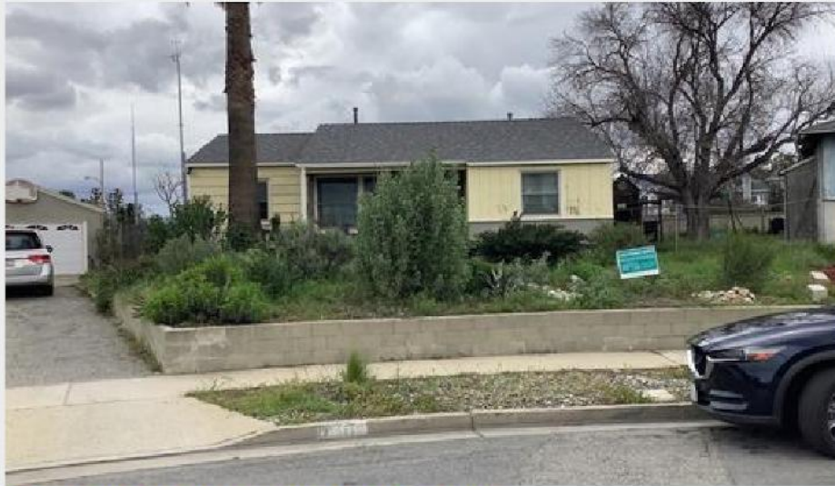
Figure 1. Front View of Main Dwelling
