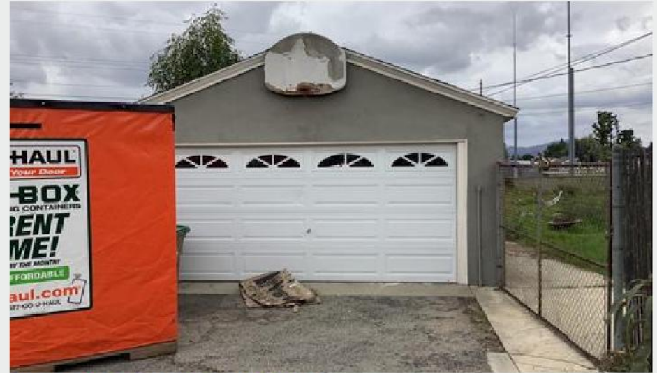
Figure 2. Front View of Garage
