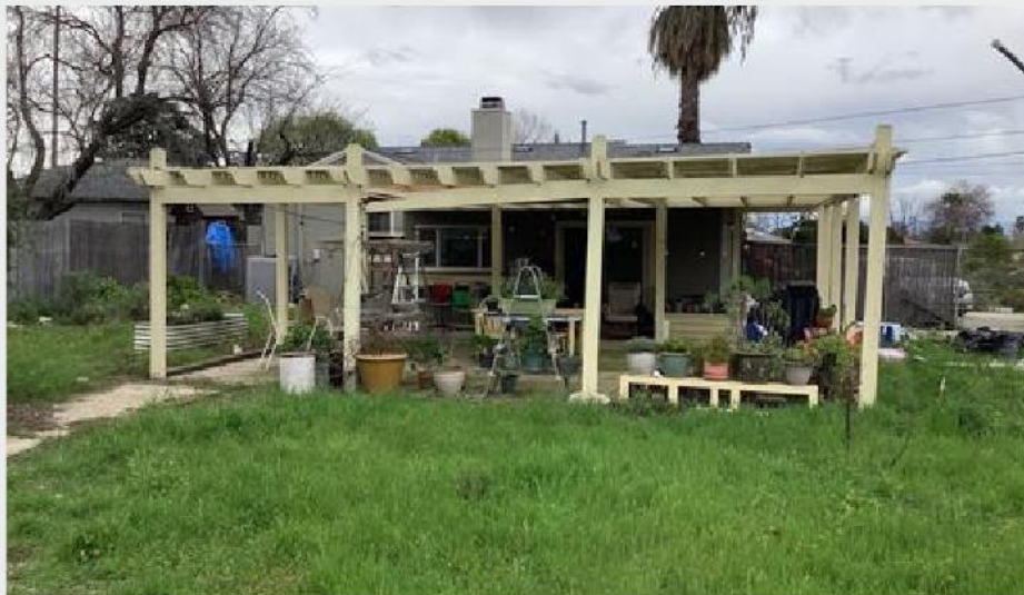
Figure 11. Pergola to be Demolished
