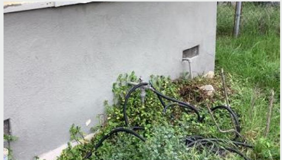
Figure 20. Main Water into Dwelling
