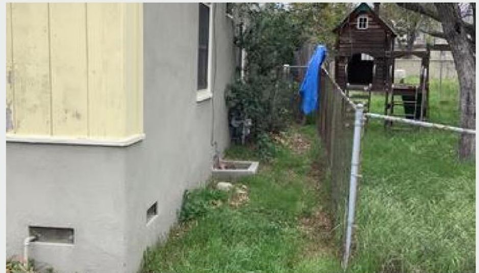
Figure 16. Nearest Sewer Point to ADU
